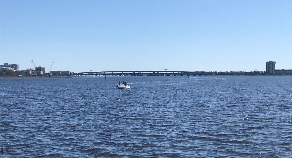
Figure 2-3. At Higgins Pier, looking downstream towards Brittlebank Park
